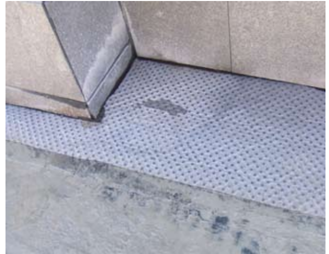
Photo 8. Drainage cell fabric under the tiling screed makes it easy to direct subterranean water to designated outlets.
