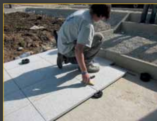
CLEAR DRAINAGE & ROOM FOR PIPES/CABLES UNDER THE TILES
