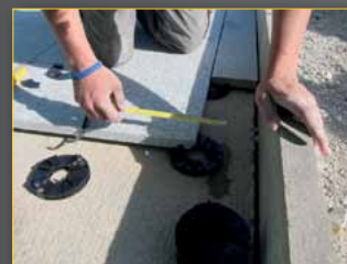
NO GLUE OR MORTAR NO GROUT NO "PICTURE FRAMING"
